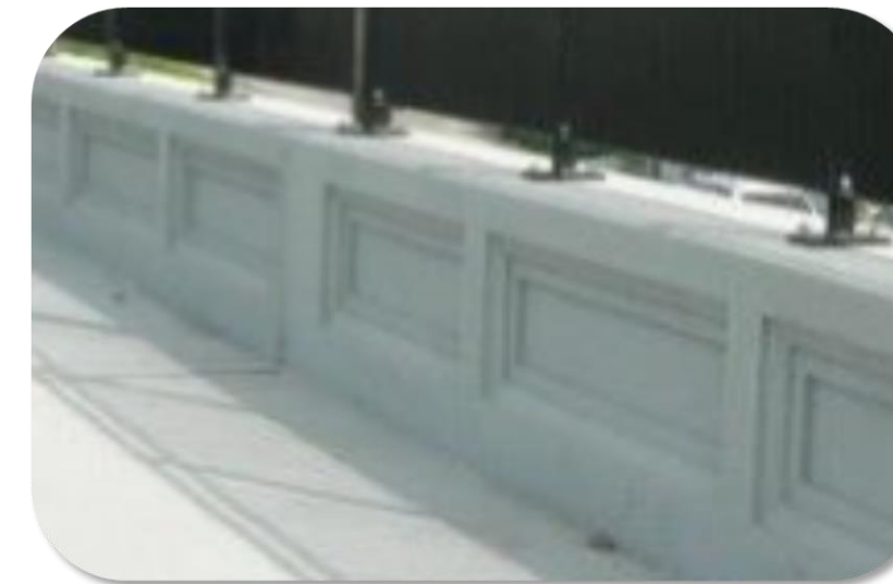
Example of formliner panels on the pedestrian side of the bridge and the highway side of the bridge.
