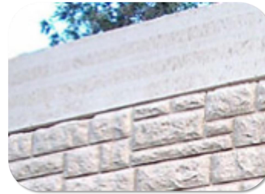
Example of ashlar formliner patterns and curved retaining walls
