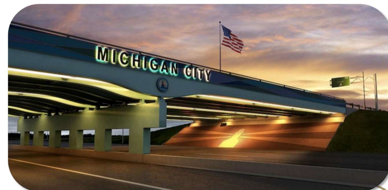
Example of girder lighting under the bridge
