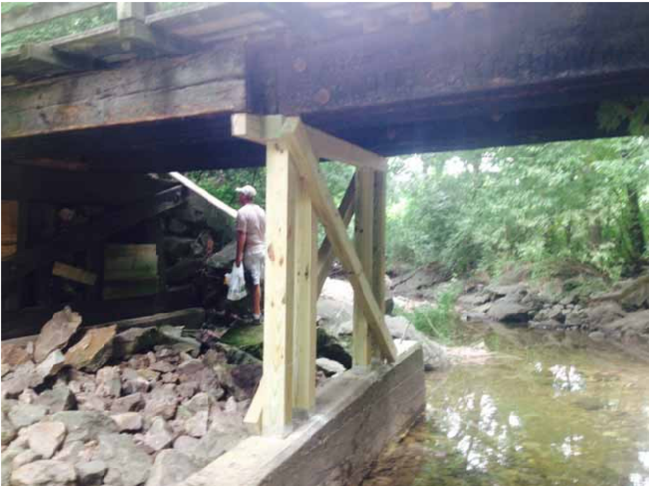
Bridge No. 5 After Temporary Repair Work
