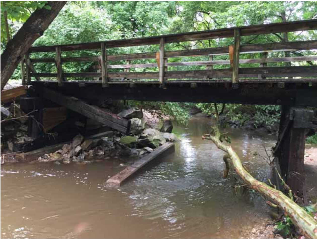
Bridge No. 5 Prior to Temporary Repair Work
