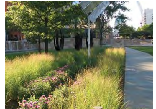
Precedent: Stormwater Bio-Swale
