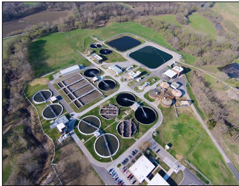
The Columbia Regional Wastewater Treatment Plant is a critical asset to effectively manage and treat wastewater from the City and surrounding area
