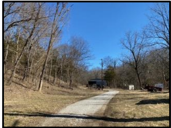
Internal access road
