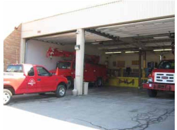
Limited conditioned space is available for essential vehicles.
