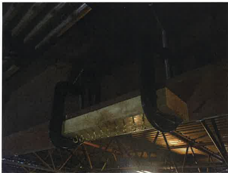
Example of anchor point mounted with C-Clamps. Ideal for Mounting on I beams.
