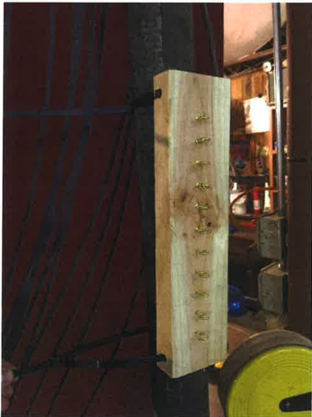
Example of Anchor point mounted with zip ties.
