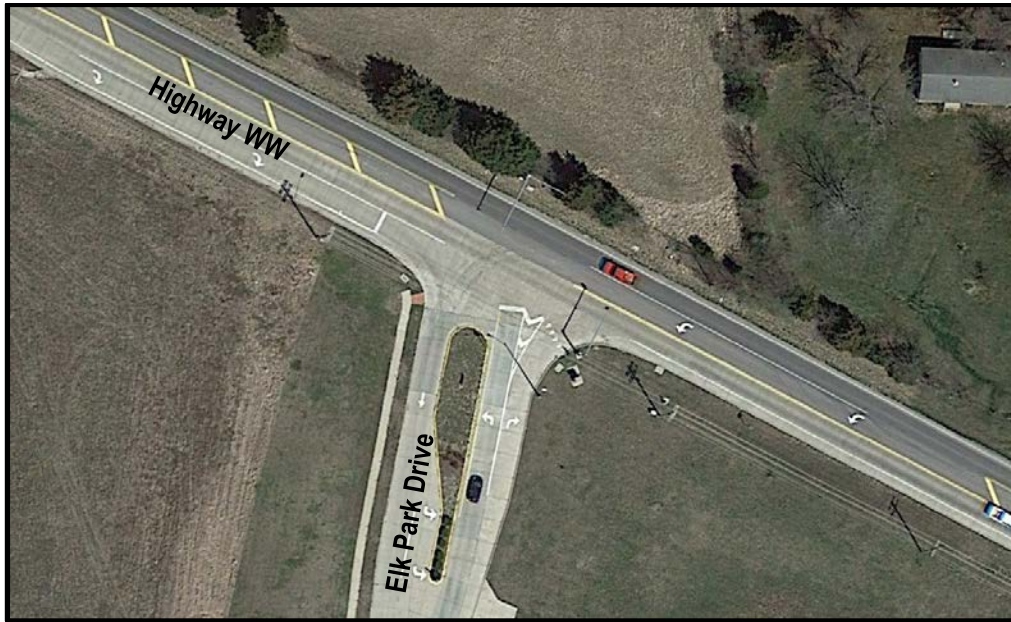
Figure 3: Highway WW at Elk Park Drive
