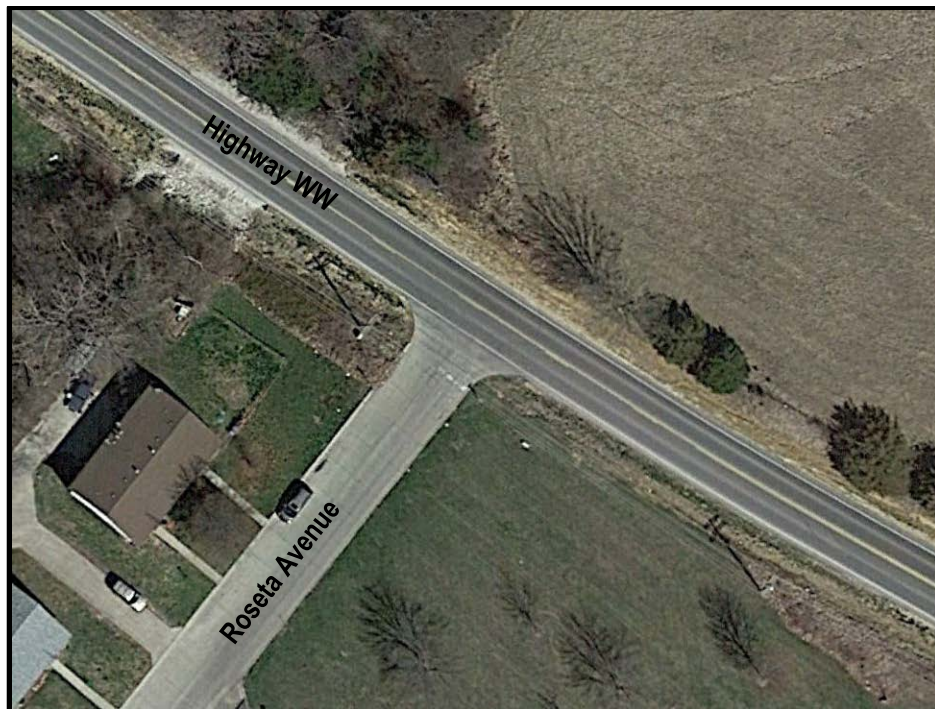
Figure 4: Highway WW at Roseta Avenue
