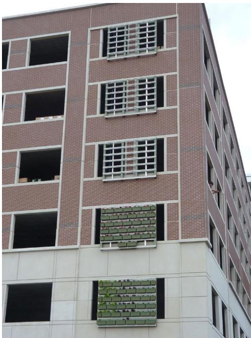
Image: LiveWall system being installed in Bloomington, IN
