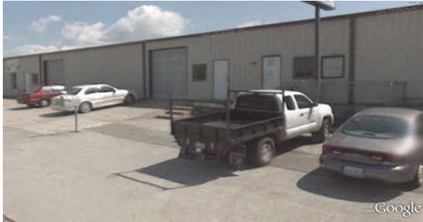
Typical view of the Lake of the Woods Warehouse Building
