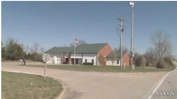
Typical view of District Station #12
