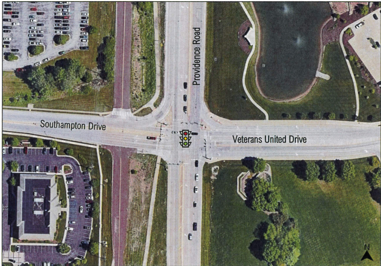
Figure 2: Aerial View of Providence Road and Southampton Drive/Veterans United Drive
