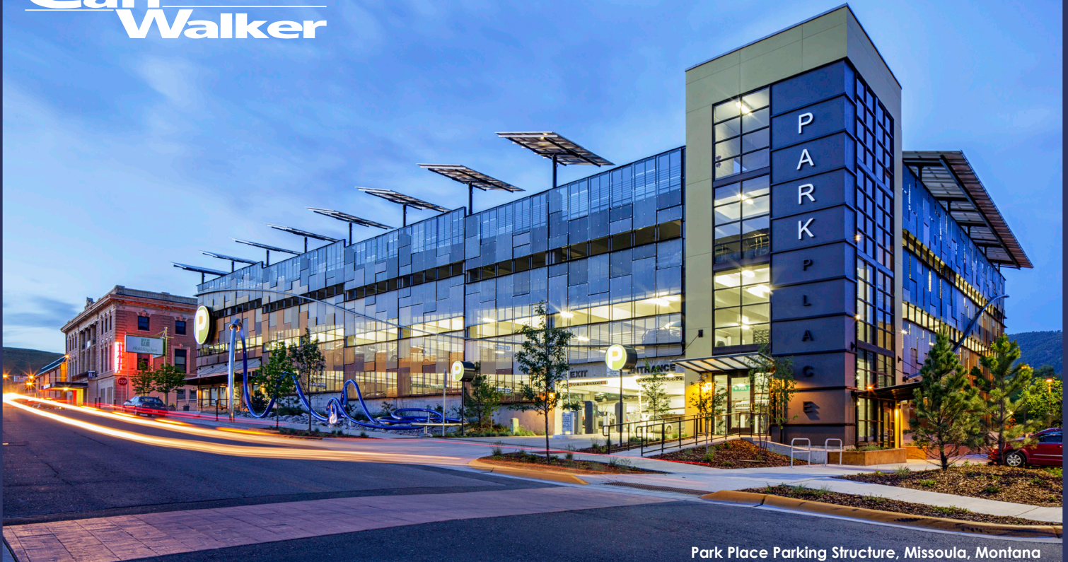
Park Place Parking Structure, Missoula, Montana
