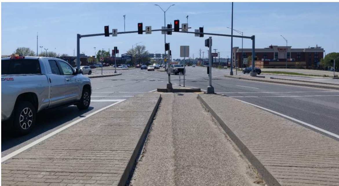
Photograph 17: Stadium Blvd DDI at I-70 (Pedestrian Bridge)
