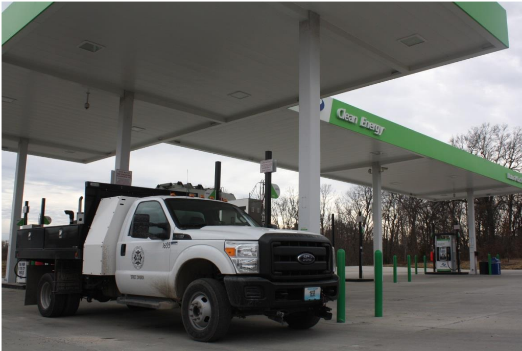
Figure 3 CNG Fueling Station
