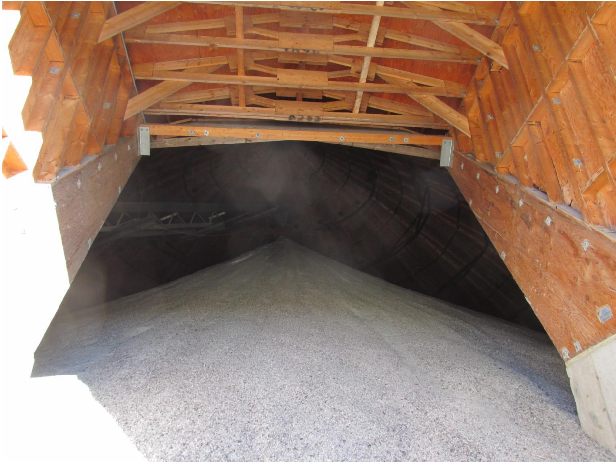
Figure 4 Salt Storage Facility
