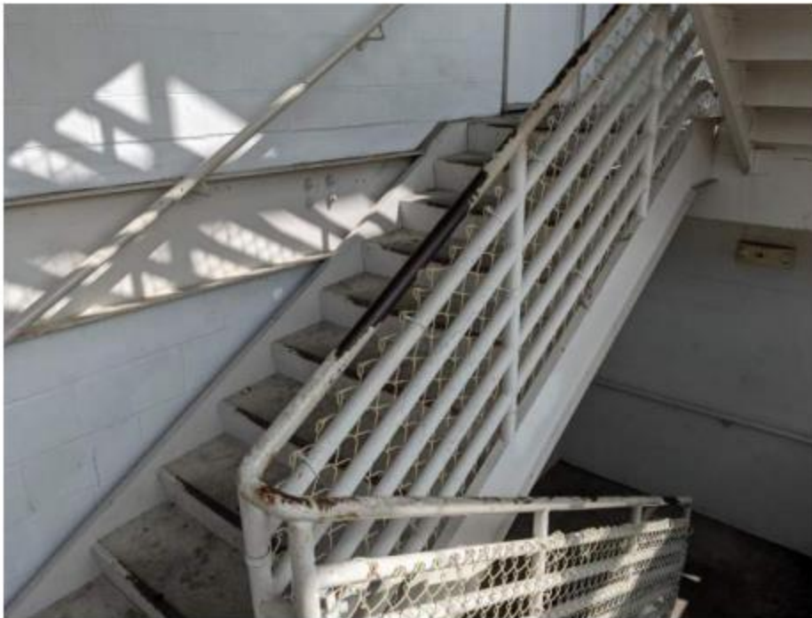
8&C -Photo 112. Typical worn paint on stair tower railings.
