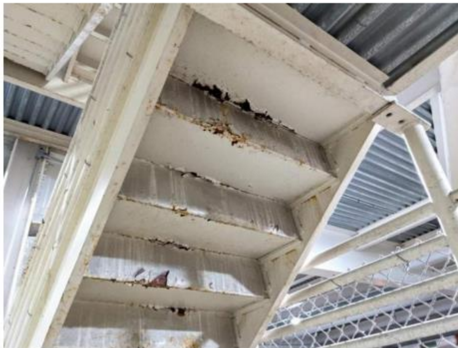
8&C -Photo 110. Underside of interior stair tower with moderate to severe corrosion.
