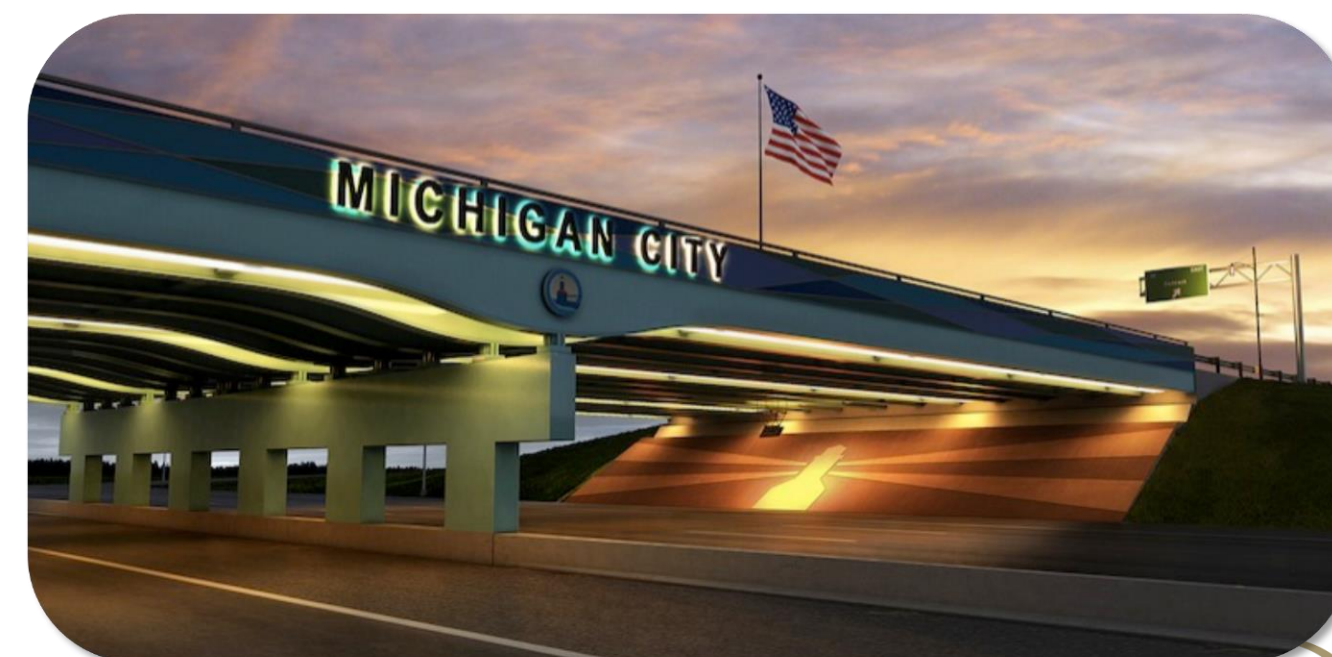
Example of girder lighting under the bridge
