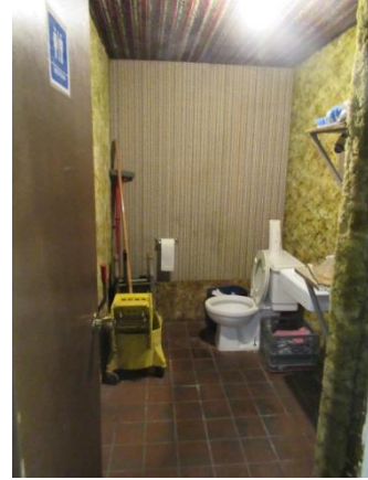
Unit A – Bathroom
