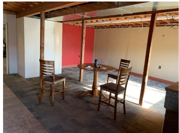
Unit A – Office
