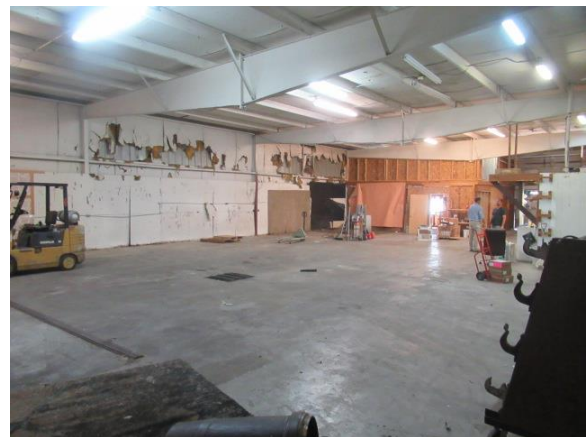
Unit A – Shop / warehouse
