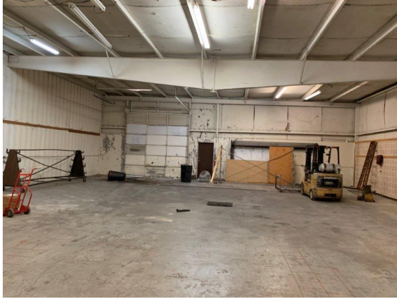
Unit A – Shop / warehouse
