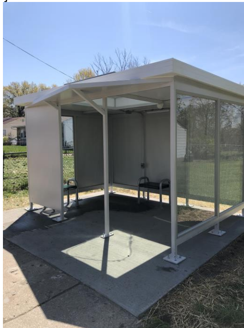
Installed bus shelter. Artwork to be installed on panel on far left.
