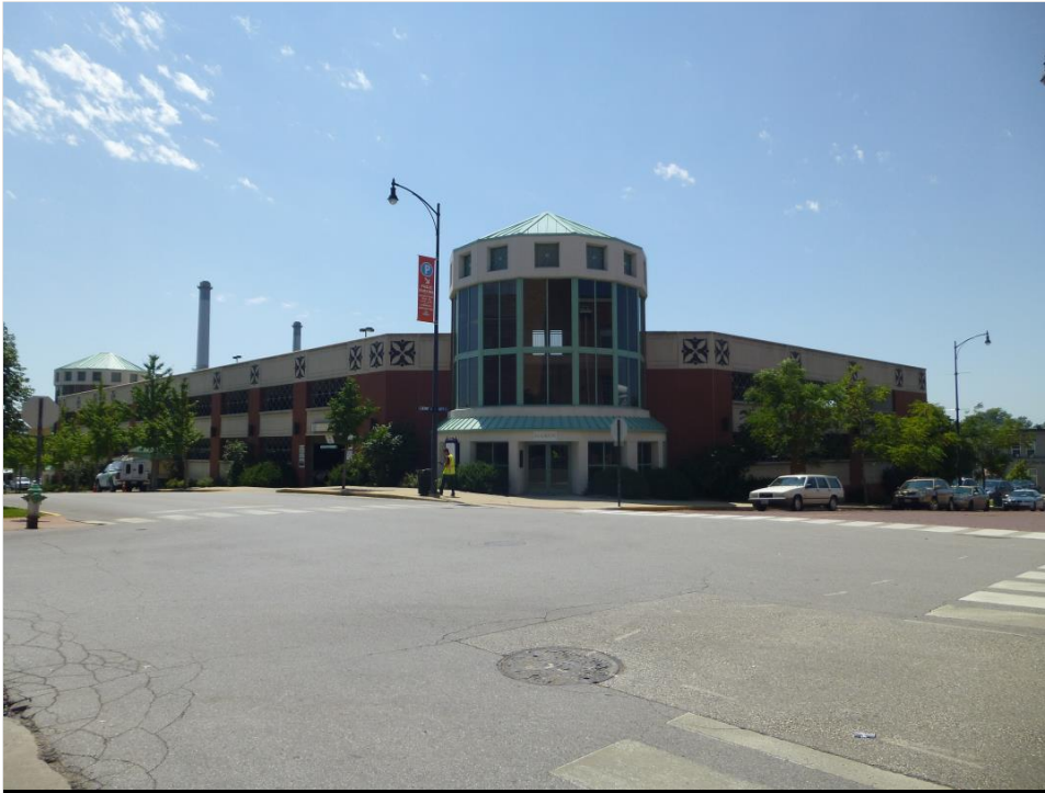
Photo 1 – North and East elevation of the parking structure.
