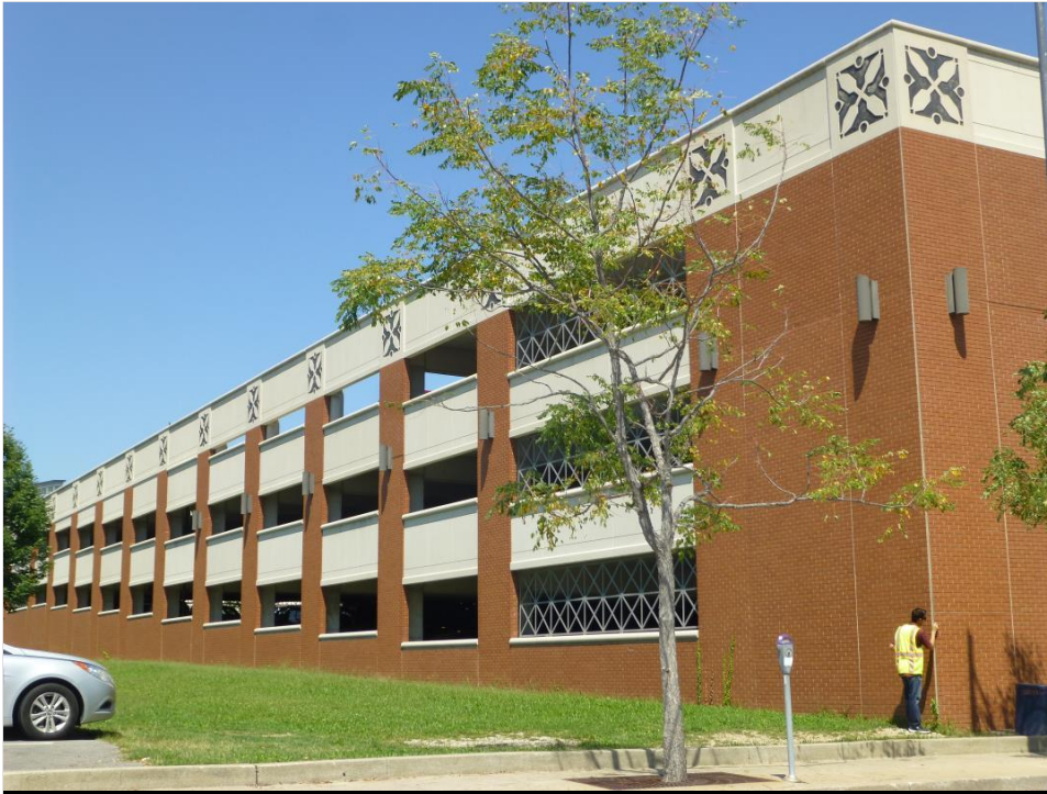
Photo 3 – West elevation of the parking structure.
