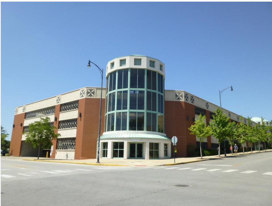
Photo 2 – South and East elevation of the parking structure.
