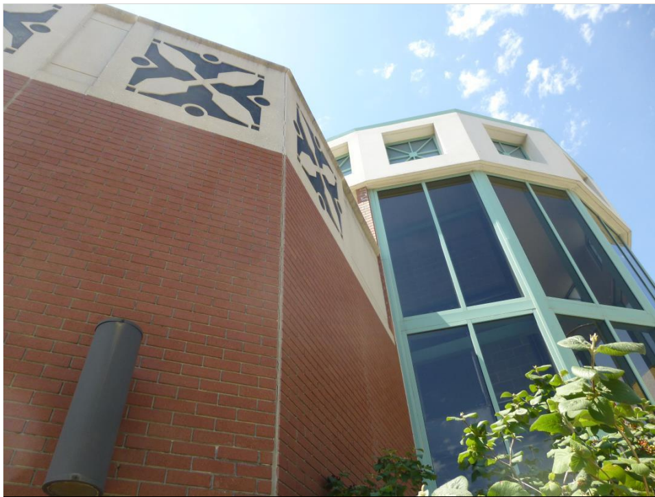
Photo 14 – View of typical vertical isolation joint installed throughout façade.
