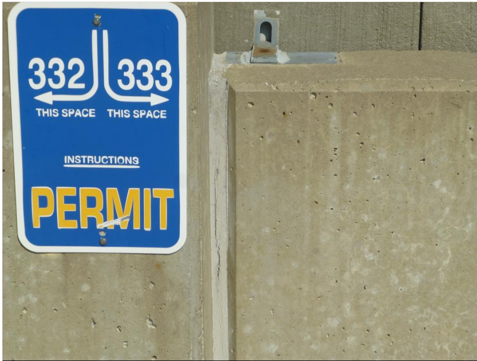
Photo 13 – Failed vertical joint sealant at stub column.
