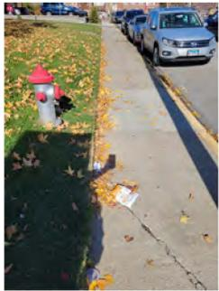
**#1: REMOVE & RECONSTRUCT SIDEWALK PANELS (18'x7').**
