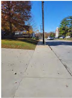
**#2: REMOVE SIDEWALK PANEL. CONSTRUCT SIDEWALK WITH INTEGRAL CURB TO WIDEN SIDEWALK AROUND UTILITY POLE (10'x7').**
