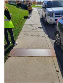
**#7: REMOVE & RECONSTRUCT SIDEWALK PANELS (35'x5').**
