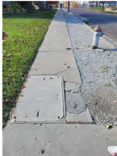
**#2: GRADE IN ADDITIONAL GRAVEL TO SIDEWALK/CURB ELEVATION. BID ALTERNATE: REMOVE GRAVEL (INCIDENTAL TO WORK), CONSTRUCT 6" SIDEWALK WITH INTEGRAL CURB.**
