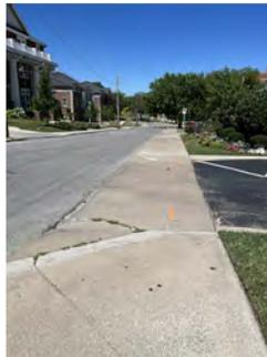
**#3: REMOVE & RECONSTRUCT DRIVEWAY APPROACH/SIDEWALK. REMOVE & RECONSTRUCT 2 SIDEWALK PANELS ON EACH SIDE OF DRIVEWAY. WARP SIDEWALK AS POSSIBLE FOR ADA.**
