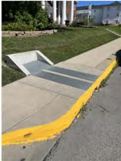
**#1: REMOVE TRENCH GRATES IN SIDEWALK & REPLACE WITH NEENAH R-4999-DX WITH TYPE D LID TO REMOVE SLIP HAZARD. SEE DETAIL ON SHEET 3.**
