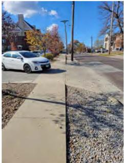
**#1: GRADE IN ADDITIONAL GRAVEL TO SIDEWALK/CURB ELEVATION. BID ALTERNATE: REMOVE GRAVEL (INCIDENTAL TO WORK), CONSTRUCT 6" SIDEWALK WITH INTEGRAL CURB.**
