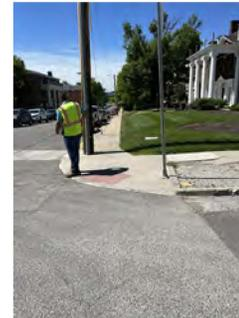
**#5: REMOVE & RECONSTRUCT CURB RAMP, SIDEWALK PANEL AROUND UTILITY BOX, 2 PANELS AROUND UTILITY POLE/BUMP OUT AROUND POLE (10'X7.5')**
