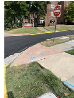
**#5: REMOVE & RECONSTRUCT CURB RAMP & 1 SIDEWALK PANEL ON EACH SIDE TO CREATE LANDING & RAMPS. REMOVE & RECONSTRUCT CURB & GUTTER. INSTALL DETECTABLE WARNING.**
