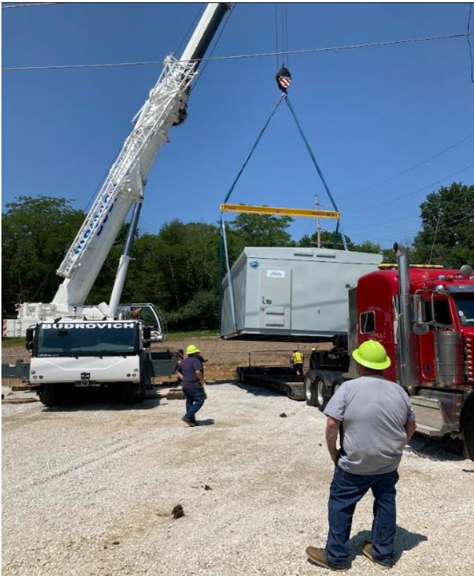
Switchgear Installation at Perche Substation for new transformer.
