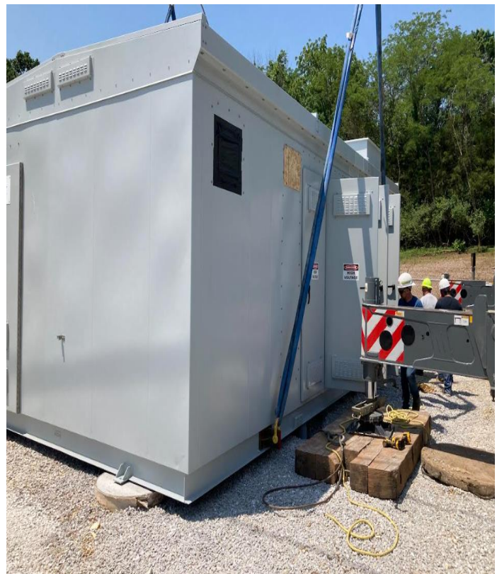
Switchgear Installation at Perche Substation for new transformer.
