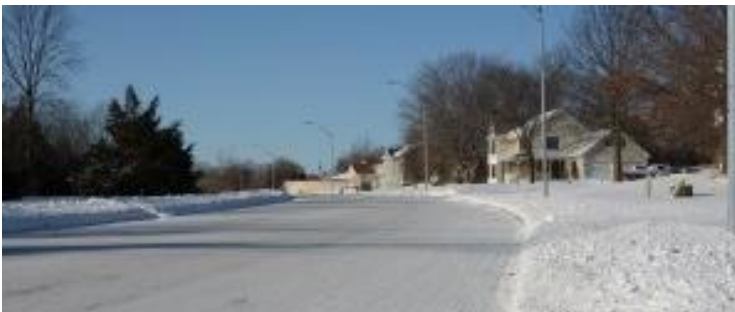
This is a second priority city street showing both driving lanes as plowed yet limited pavement visible. This road meets the definition of passable. Lack of bare wheel path most likely to occur during times of extreme cold (10 degrees or less).
