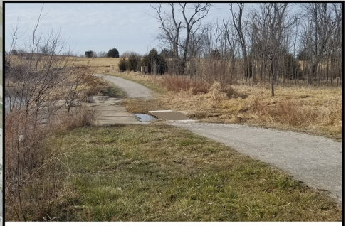
EXISTING LOW WATER CROSSING
