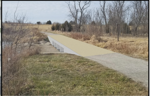
PROPOSED LOW WATER CROSSING 16 feet wide to provide a 8 foot wide trail with 4 foot wide shoulders and curbing Approximately 60 feet long
