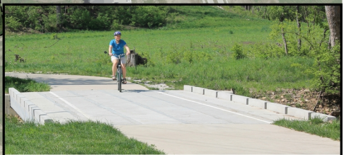
SIMILAR LOW WATER CROSSING Proposed Low Water Crossing will have a similar deck design as the bridges on the County House Trail
