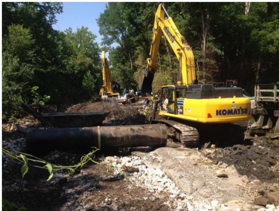
Flat Branch Sewer Relief Project
