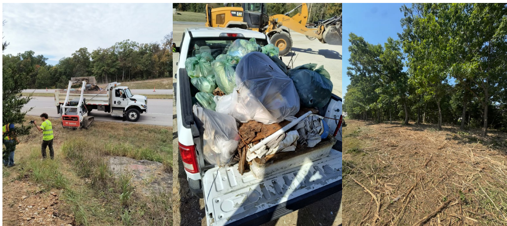
Figures 15-17. City of Columbia cleanup: Collecting and hauling waste and clearing areas with a forestry head.
