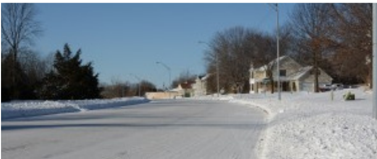
This is a second priority city street showing both driving lanes as plowed yet limited pavement visible. This road meets the definition of passable. Lack of bare wheel path most likely to occur during times of extreme cold (10 degrees or less).
