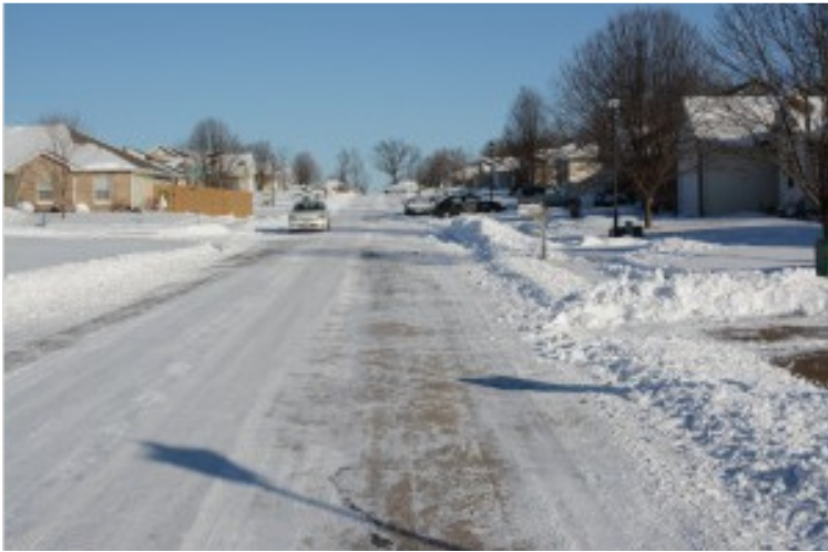
This is a city street showing both driving lanes as plowed where patches of pavement are visible. This road meets the definition of passable.
