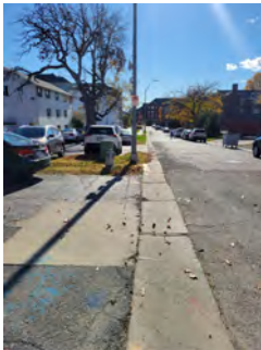
#1: CONSTRUCT NEW SIDEWALK AND DRIVEWAY APPROACHES.
