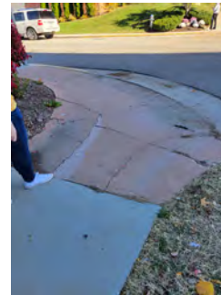
#5: REMOVE & RECONSTRUCT CURB RAMP & NORTH SIDE SIDEWALK PANELS TO CREATE SMALLER LANDING & RAMPS. REMOVE & RECONSTRUCT CURB & GUTTER. INSTALL DETECTABLE WARNING.
