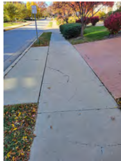
#2: REMOVE & RECONSTRUCT SIDEWALK PANELS (28'x5').
