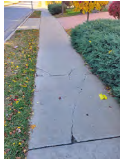
#3: REMOVE & RECONSTRUCT SIDEWALK PANELS (10'x5').
