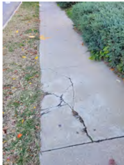
#1: REMOVE & RECONSTRUCT SIDEWALK PANELS (11'x5').
