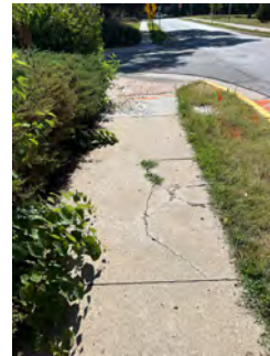
#4: REMOVE & RECONSTRUCT SIDEWALK PANELS (5'x5').
