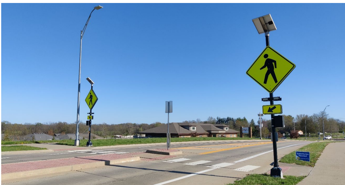
Photograph 8: Scott Blvd South of Abbington Terrace (RRFB)
