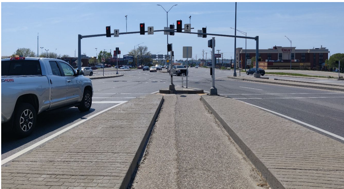
Photograph 17: Stadium Blvd DDI at I-70 (Pedestrian Bridge)
