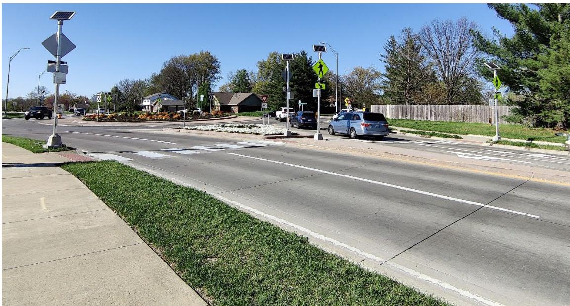
Photograph 7: Forum Blvd & Green Meadows (RRFB at Roundabout)
