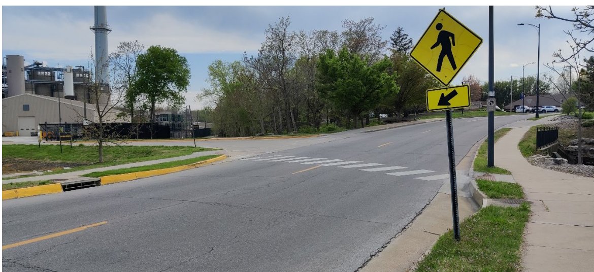
Photograph 14: Elm Near Providence (unsignalized crossing)
