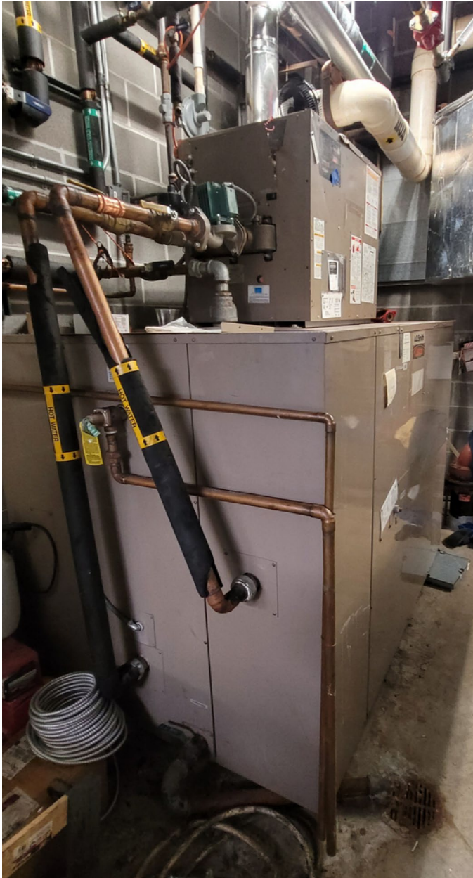
Domestic Hot Water Heater Replacement
