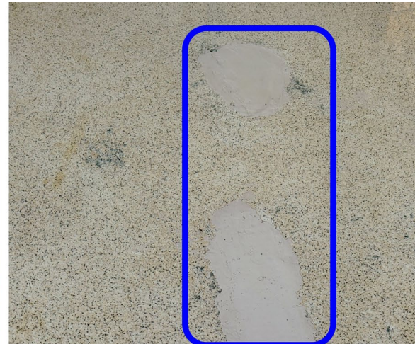
Water Play Structure Area Aggregate Flooring Replacement
