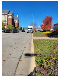
#2: CONSTRUCT NEW SIDEWALK AND DRIVEWAY APPROACHES.
