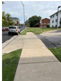
#3: REMOVE & RECONSTRUCT DRIVEWAY APPROACH/SIDEWALK (34'X5'), REMOVE & RECONSTRUCT CURB & GUTTER.
