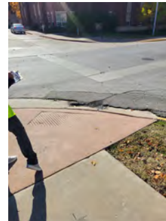
#4: REMOVE & RECONSTRUCT CURB RAMP & 2 SIDEWALK PANEL ON EACH SIDE TO CREATE LANDING & RAMPS. REMOVE & RECONSTRUCT CURB & GUTTER. INSTALL DETECTABLE WARNING. SEE SHEET 11.
