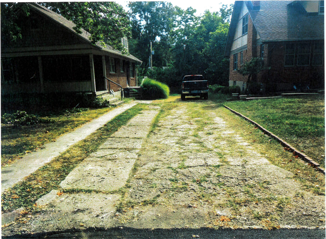
210 Edgewood Avenue (on left), recent photos of shared driveway from street
