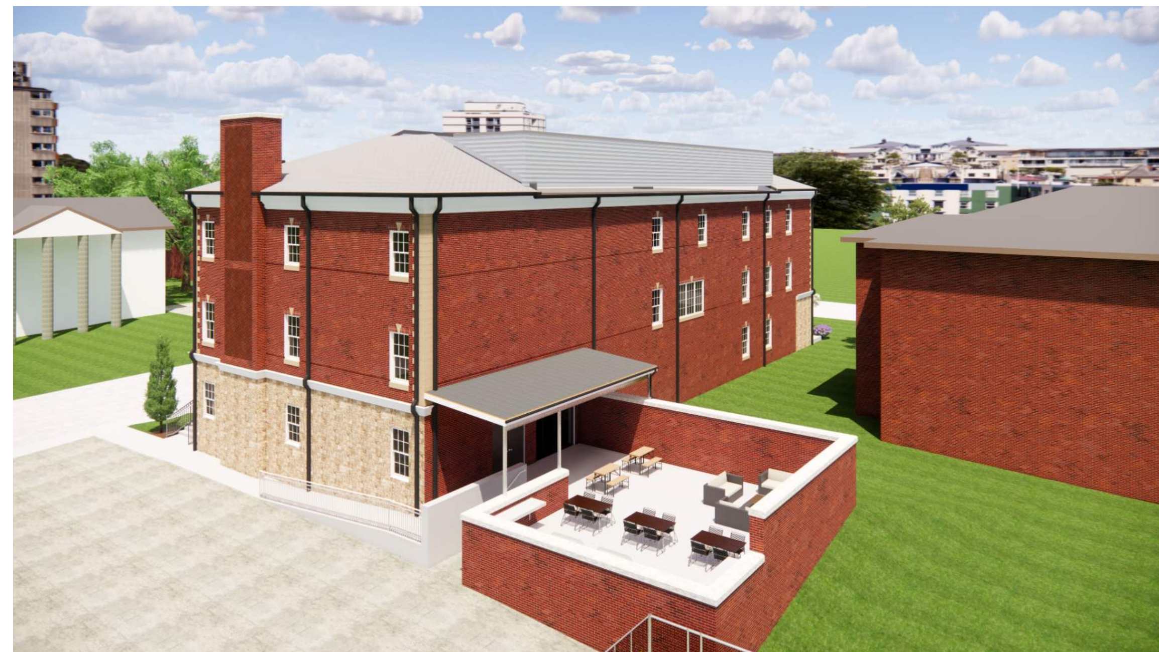
03 ELEVATED - FROM SE
