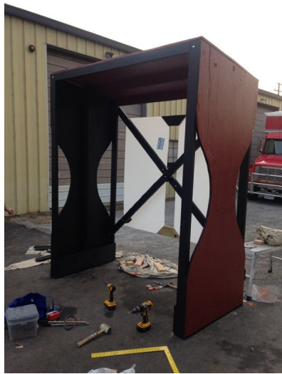
Examples of Bus Shelters installed during T/F 2017
