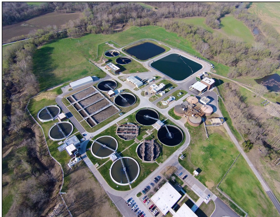
Figure 1. Aerial View of the Columbia Regional Wastewater Treatment Plant.
