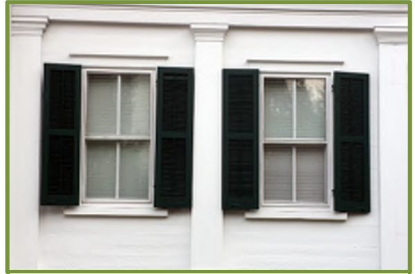
The windows on this 1848 house retain their original shutters and also incorporate exterior storm windows mounted so they do not alter the historic character of the windows.
