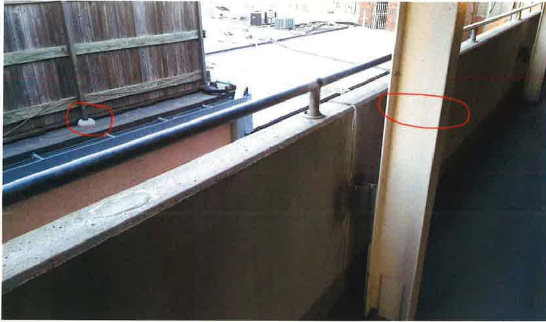
Taken from inside the parking garage, looking out onto alley.
