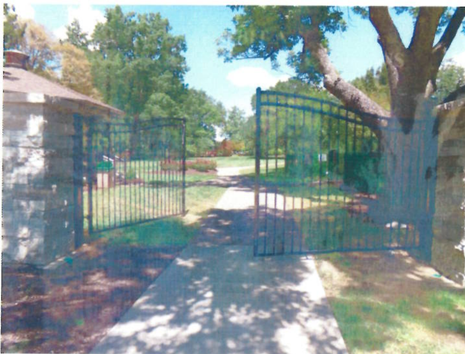
Photo 1: New Gate on South Side of Gardens
