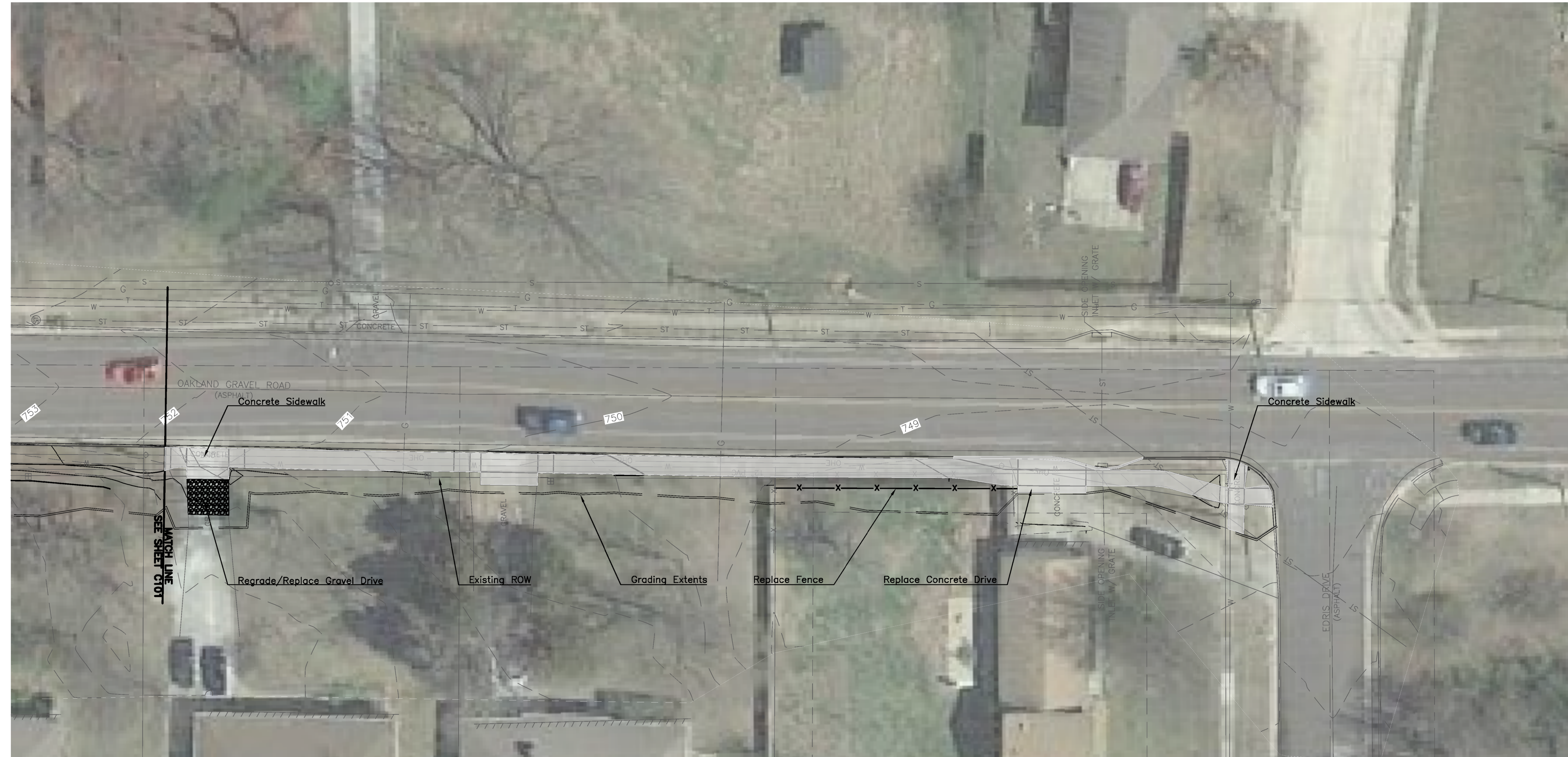
SOUTH END OF PROJECT SITE
