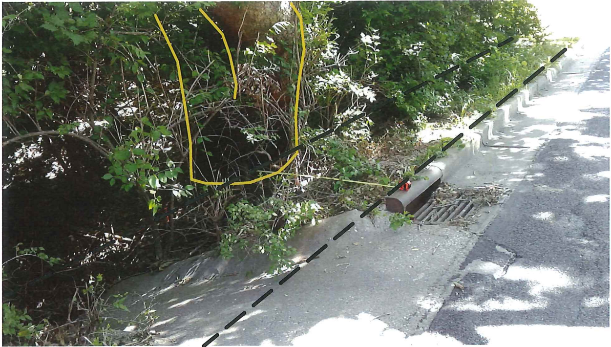
PICTURE 5: LOOKING NORTHEAST - SIDEWALK AT INLET
