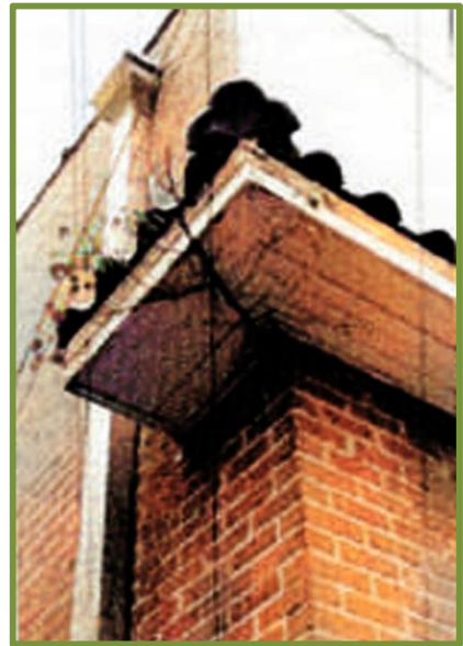
If buildings and their individual components are not maintained regularly, deterioration will surely follow. In the photo above, dirt has accumulated in the gutter, encouraging the growth of unwanted and potentially damaging plant material.
