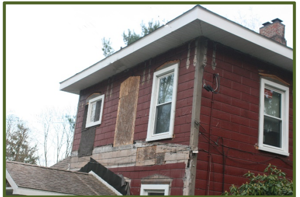
This 1890's house has suffered from the original windows being removed, along with their associated trim, including brackets, and other windows being altered.
