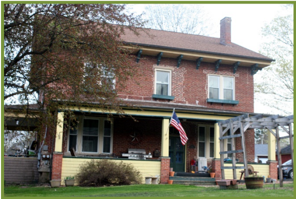
The windows on this 19th-century house had been altered significantly and the house had been previously painted. It was ultimately stripped of the paint, leaving clean evidence of the alterations. It should have been repainted rather than stripped.
