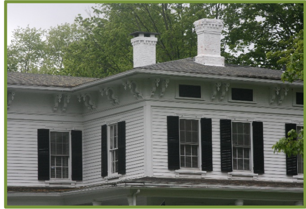
Roof forms and trim, including the bracketed cornice with "eyebrow" windows and the corbeled brick chimneys should also be retained.
