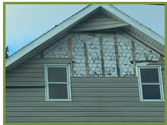
As shown above, when non-historic siding is installed, it always covers historic finishes, some of which may be decorative and may add to the architectural character of the building.
