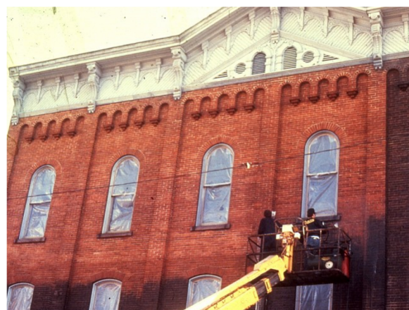
The cleaning of this previously-unpainted 1880s building demonstrates the dramatic visual effect of properly executed masonry cleaning. Using an environmentally-acceptable cleaning solution and a low-pressure water rinse, the surfaces were cleaned without any repointing being necessary.
