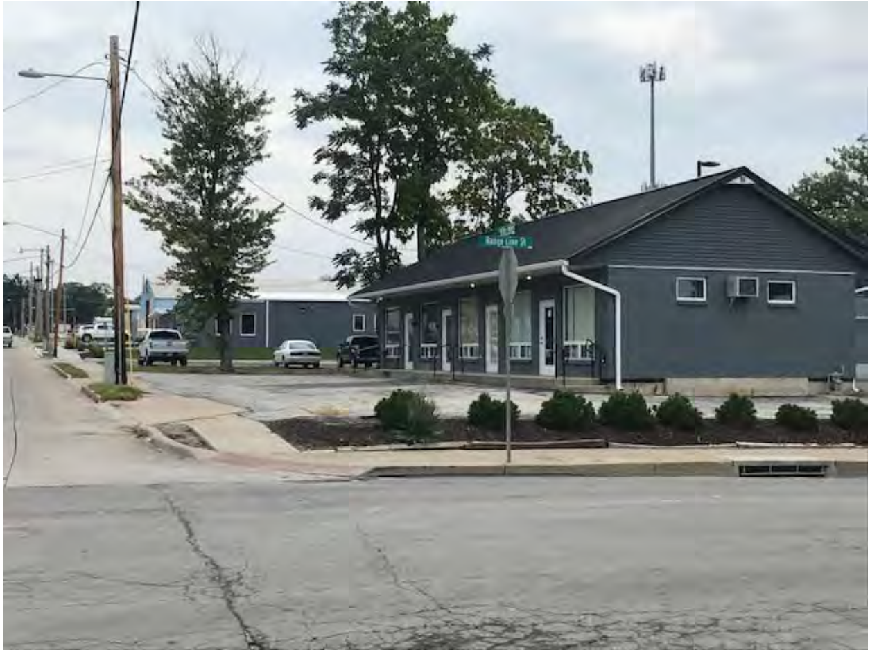
Columbia College adaptive reuse of existing heavy commercial/industrial facilities.
