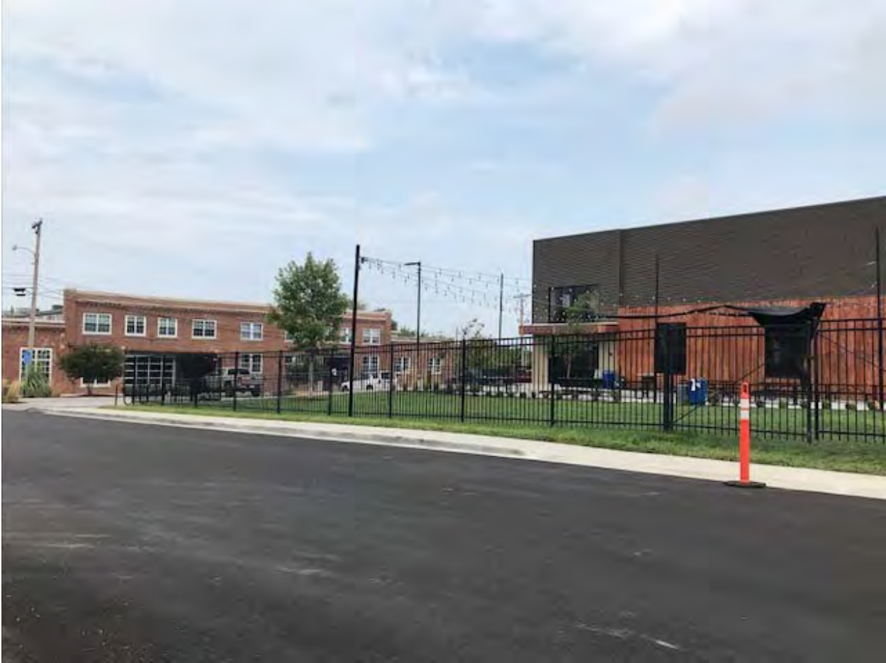
Wright Brothers Mule Barn with modern redevelopment/remodel (Logboat Brewery) in foreground.
