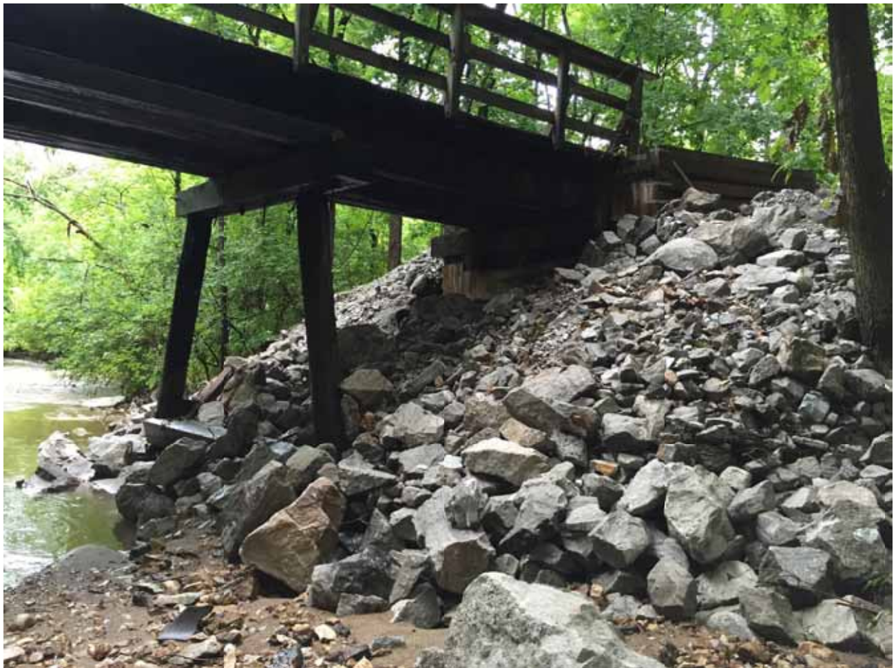
Bridge No. 7 After Temporary Repair Work in 2015
