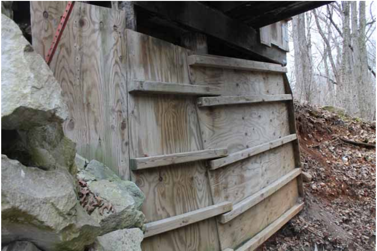
Bridge No. 7 Temporary Repair Prior to Rip-Rap
