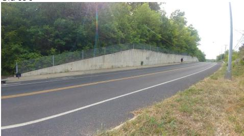
The entirety of the retaining wall is approximately 450ft long and 9ft tall. The wall is untreated concrete and is intact with no cracks. There has been unmitigated graffiti on this wall for at least four years and community murals have a proven history of helping to deter graffiti. The mural will occupy the central third of the wall with some graphic elements on the sides of the design to ensure visual cohesion of the entire wall. It is outdoors on a public street and is therefore accessible.
