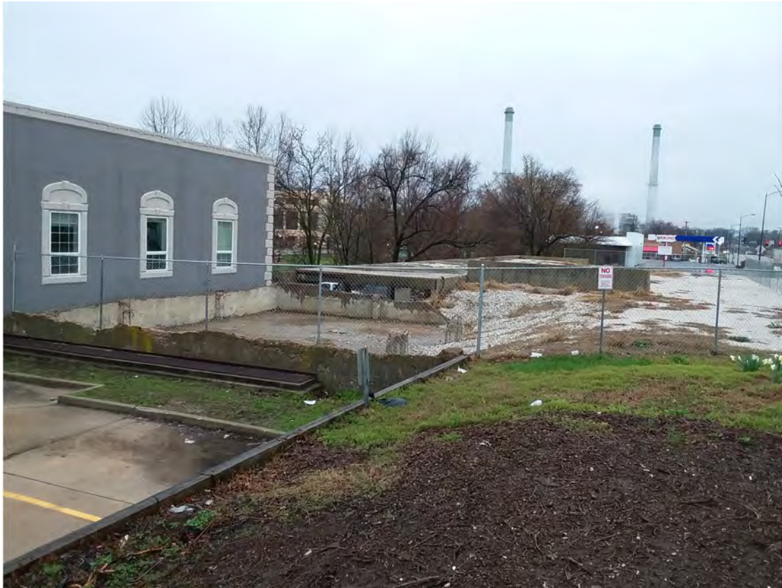
View from parking area to the south
