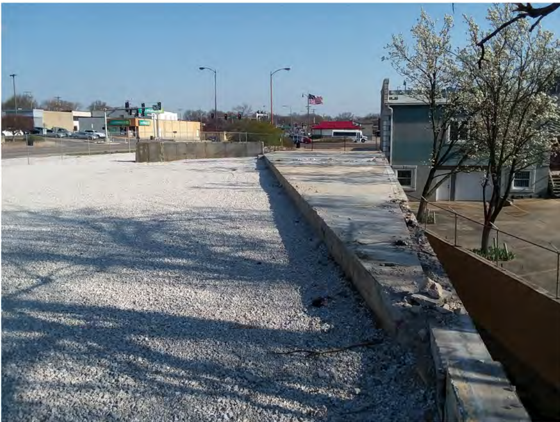
View from the Cherry St ROW to the north
