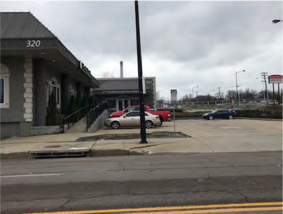
Light pole and storm inlet would need to be relocated if Option 3 is chosen.
