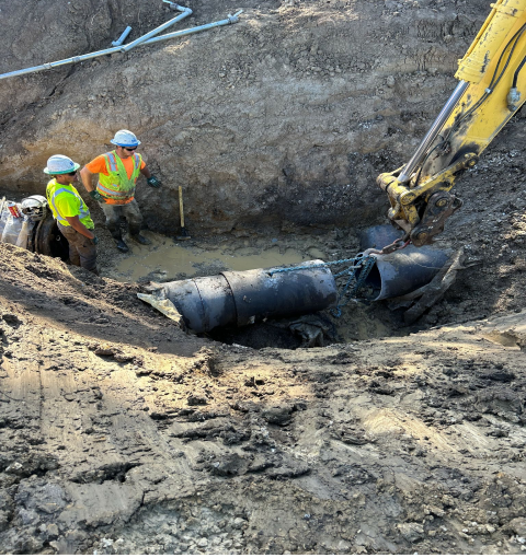
Picture top left: sewer maintenance
