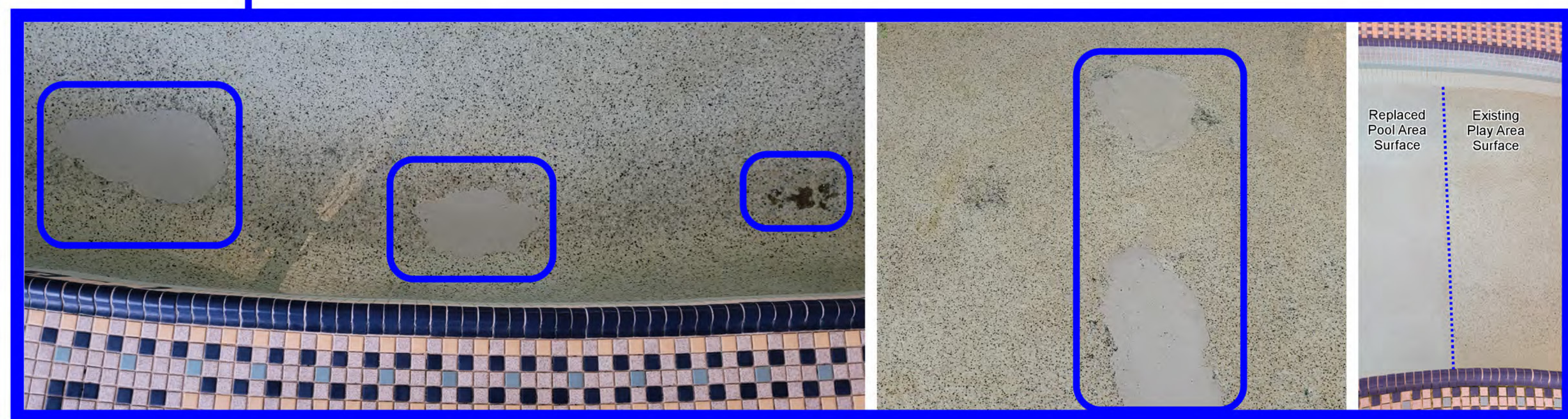
Water Play Structure Area Aggregate Flooring Replacement
