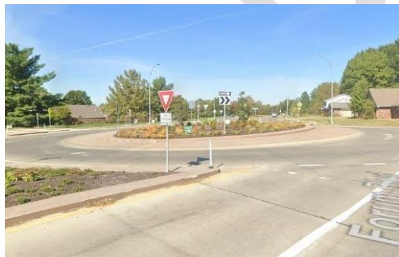
Roundabouts have emerged as an effective traffic control strategy, providing multiple benefits in terms of safety, traffic flow, and environmental impact. According to the Federal Highway Administration (FHWA), modern roundabouts improve intersection safety by reducing vehicle speeds, minimizing conflict points, and creating a counterclockwise flow around a central island. These design features significantly lower the risk of severe crashes, reducing fatal
