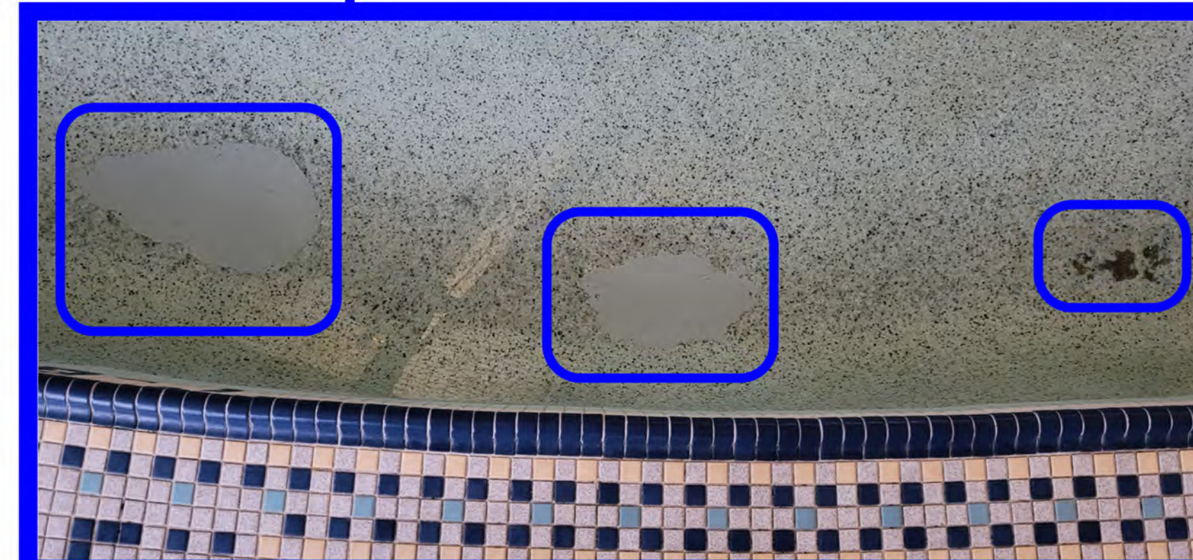
Water Play Structure Area Aggregate Flooring Replacement
