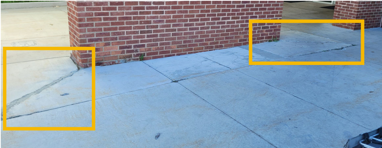
ARC Entry Area
