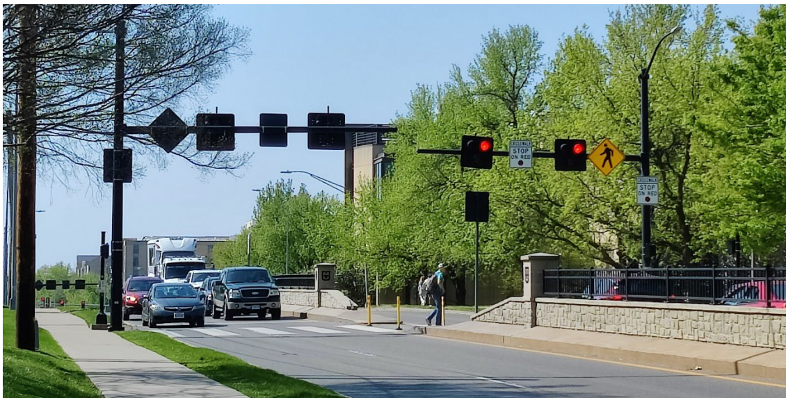
Photograph 2: S College Ave between Wilson Ave & Rosemary Ln (HAWK)
