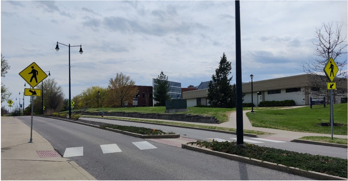
Photograph 19: Rangeline St South of Wilkes Blvd (Unsignalized Crossing)
