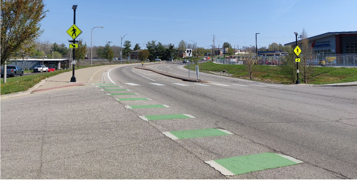
Photograph 9: S Old 63 & Access Rd (RRFB with Bike Lane)
