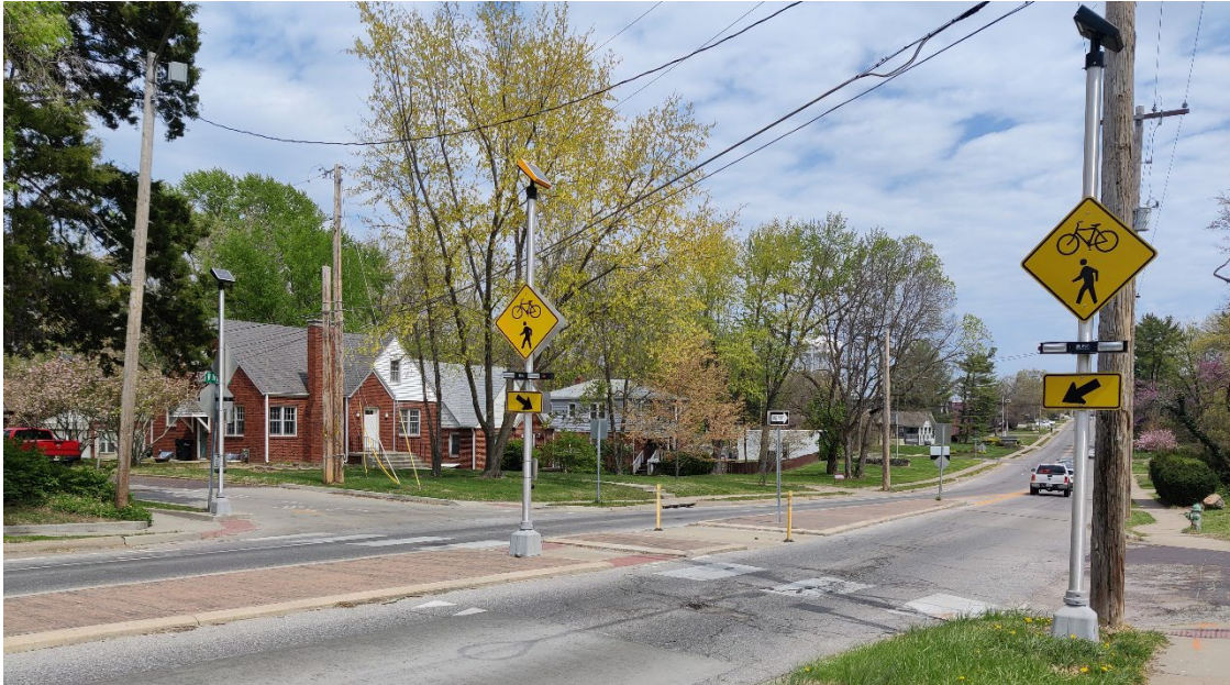
Photograph 1: W Broadway & Edgewood Ave (RRFB & Bike Boulevard)
