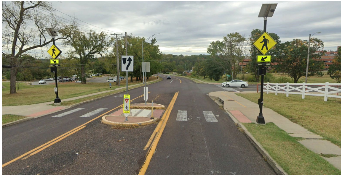
Photograph 6: Old 63 & E Walnut (RRFB on Two-Lane Road with Median)
