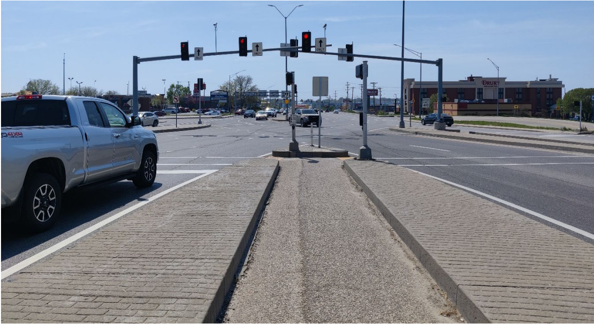
Photograph 17: Stadium Blvd DDI at I-70 (Pedestrian Bridge)
