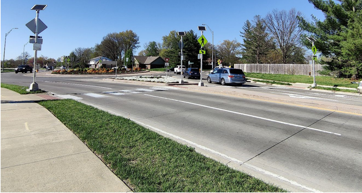
Photograph 7: Forum Blvd & Green Meadows (RRFB at Roundabout)
