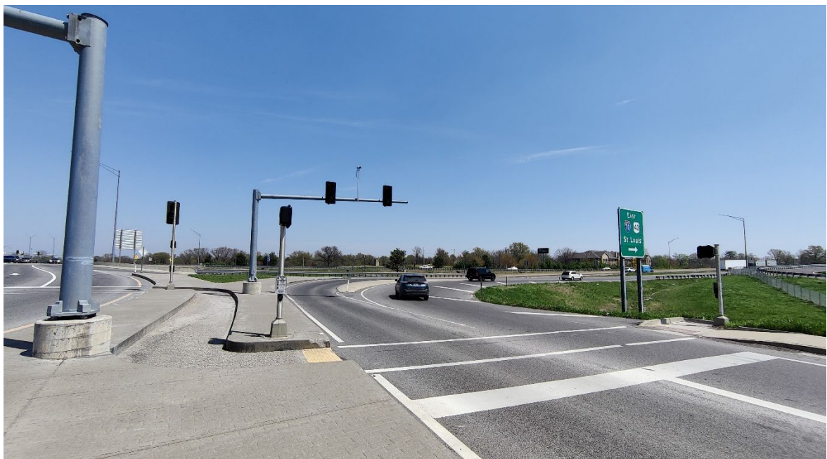
Photograph 16: Stadium Blvd DDI at I-70
