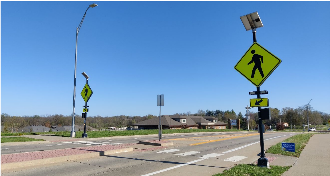
Photograph 8: Scott Blvd South of Abbington Terrace (RRFB)
